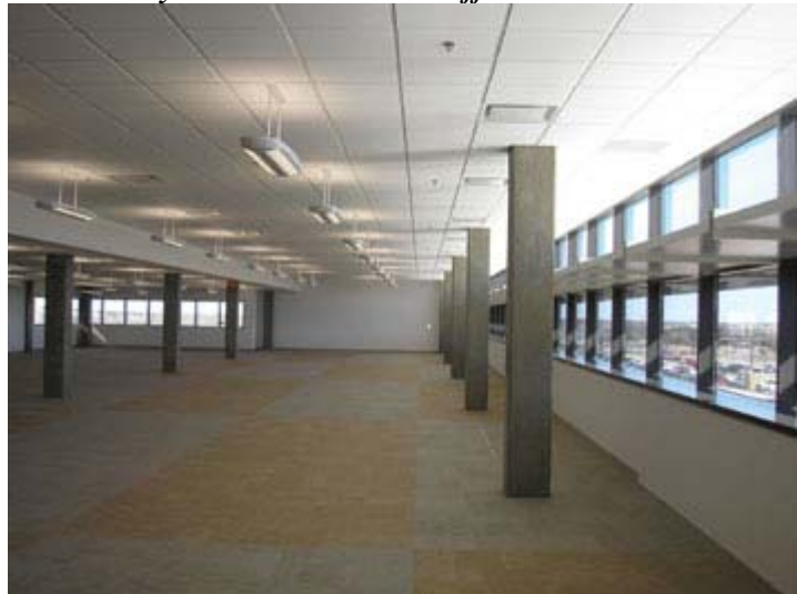
The white roof of the RFAB (above) under construction in Richardson, Texas, reflects away some 85 percent of incoming sunlight, reducing cooling loads. Daylight reflected off of window shelves in the administrative wing (below) reduces the need for artificial lighting, while the Ergolights hanging from the ceiling are designed with sensors and will shut off automatically when no one is in the office.
