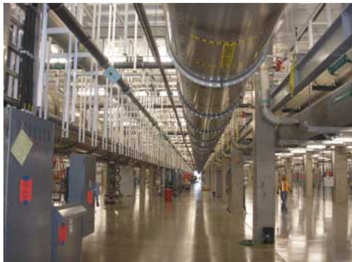
These long, straight ducts and pipes below the clean rooms carry utilities and waste more efficiently than smaller, curved pipes
