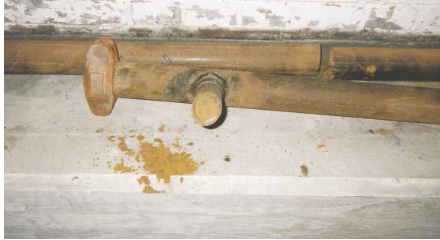
PHOTO 1. Pipe with significant scale buildup.
