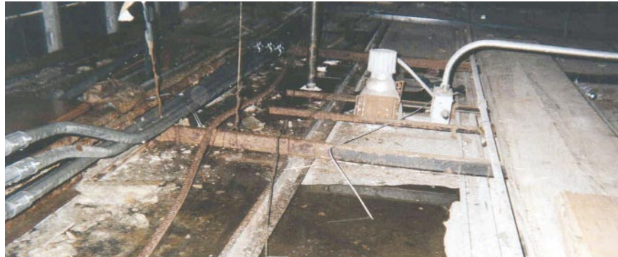
PHOTO 2. Scale buildup in this pipe led to freeze and pipe burst.
