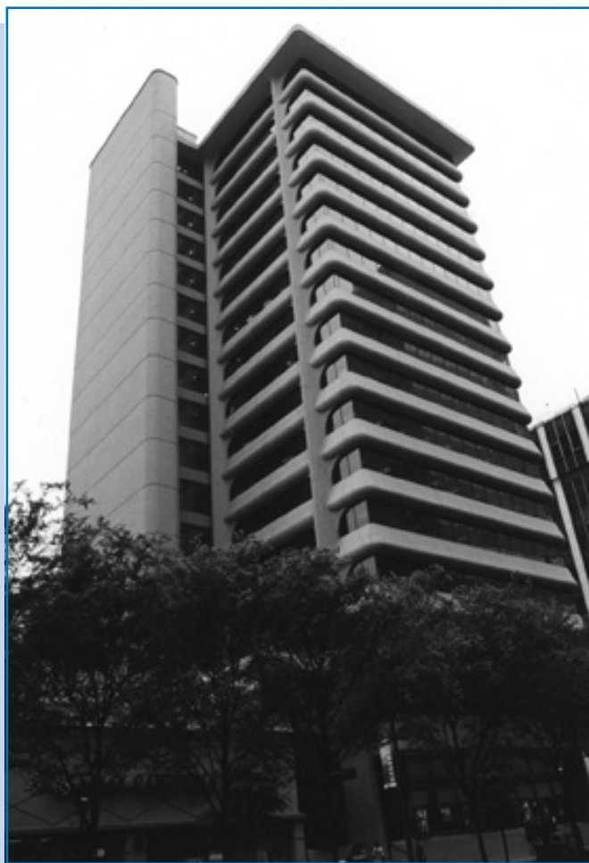
Five Points Plaza Building
